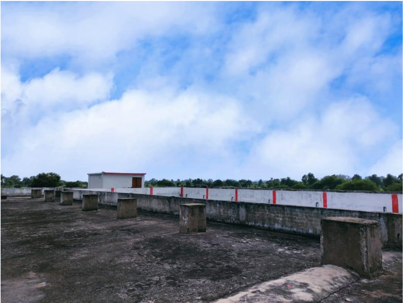
Figure - Roof of facility
