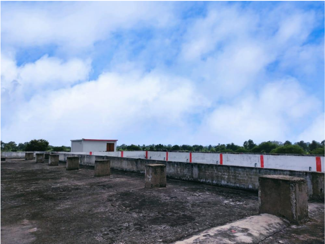
Figure - Roof of facility
