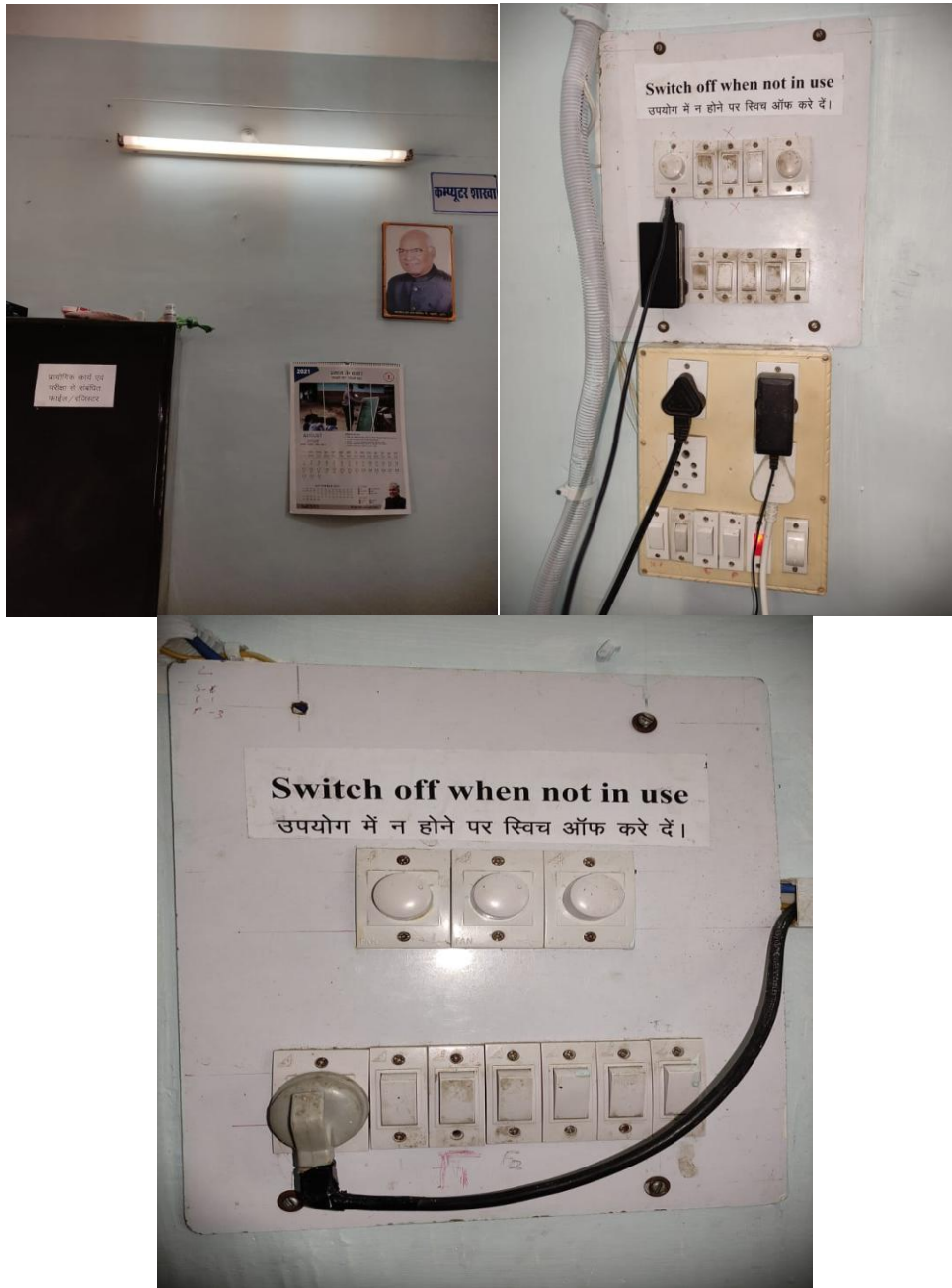
Figure - Fluorescent tubes installed in facility
